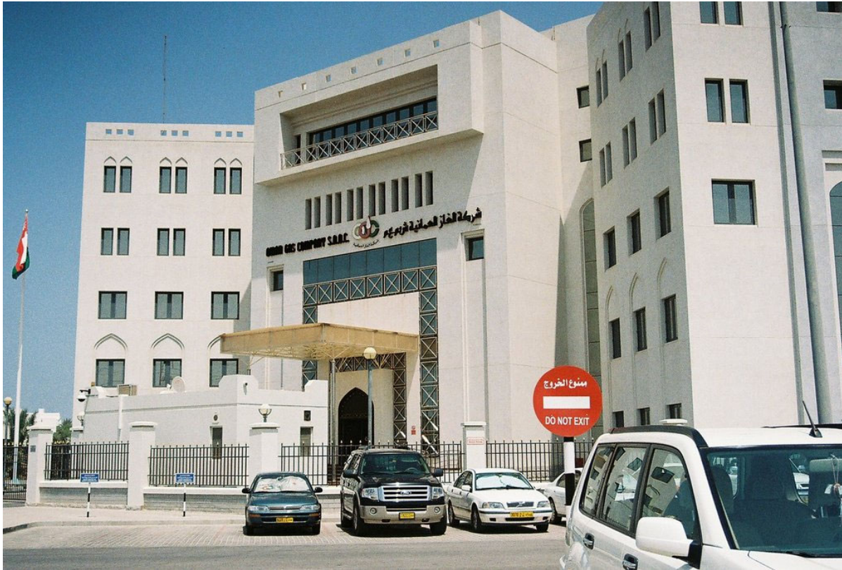
Oman Gas Company Photo by Flow Research
